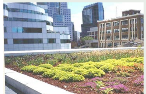
Green Roof at Mountain Equipment Co-op in Toronto
